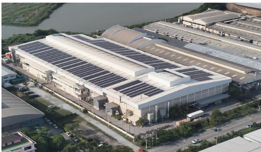
Figure 3. On-site PPA example
